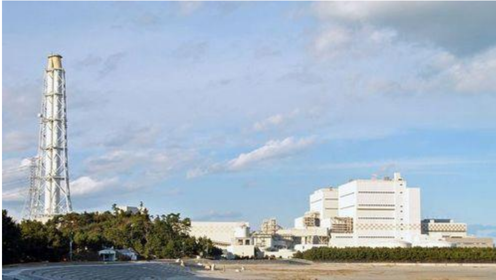
Haramachi thermal power plant Photo by Kuha455405 Some Rights Reserved.
